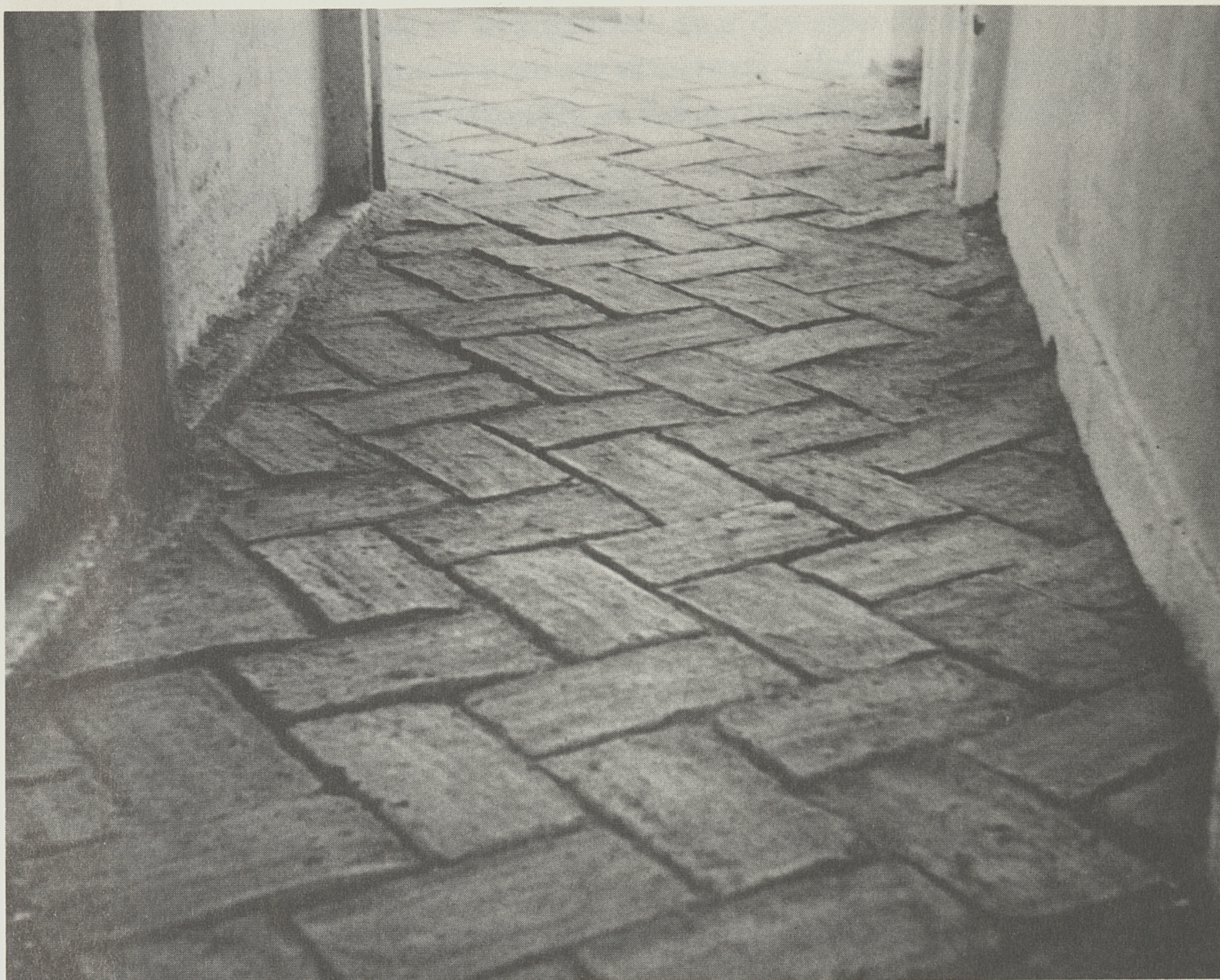
Brick Floor in Arcade (low-cost experimental housing, Mexicali)
