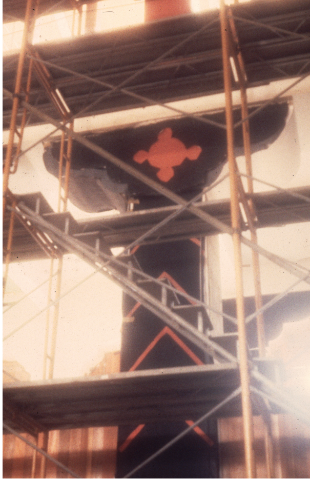
A mockup, in painted paper, of the plaster surface that was to be put on the great hall columns
