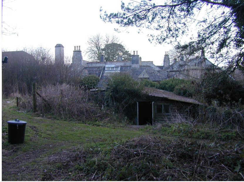
Roofs from the back
