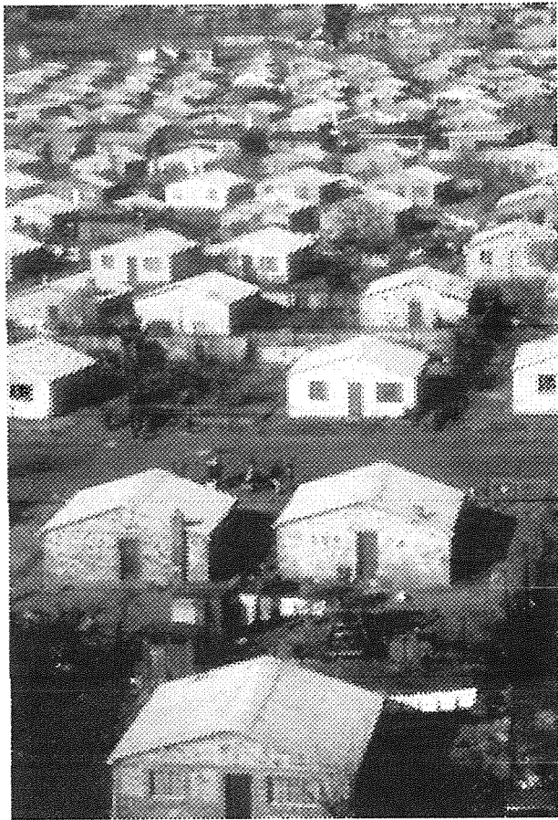
Right: Housing in Soweto
