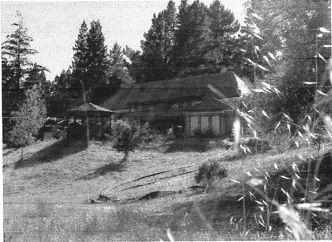
The Sanders house – the long hulk of the house and roof in the landscape
