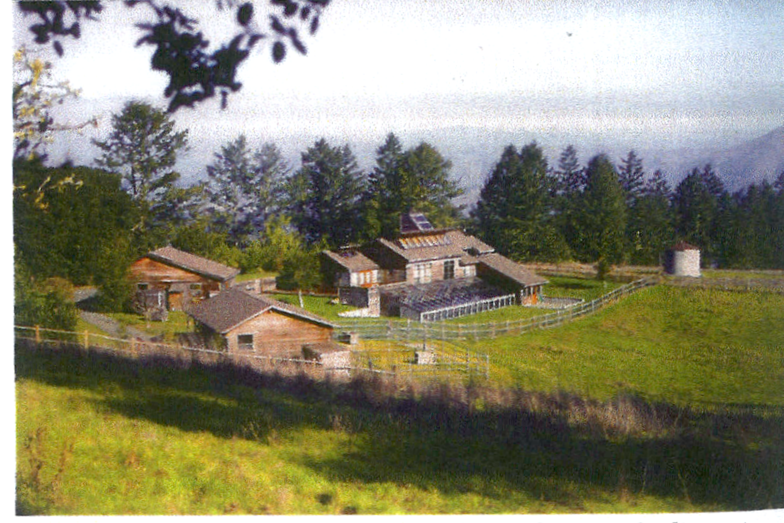
Figures 16 & 17: Johnson I House – Thermal mass of adjacent swimming pool
