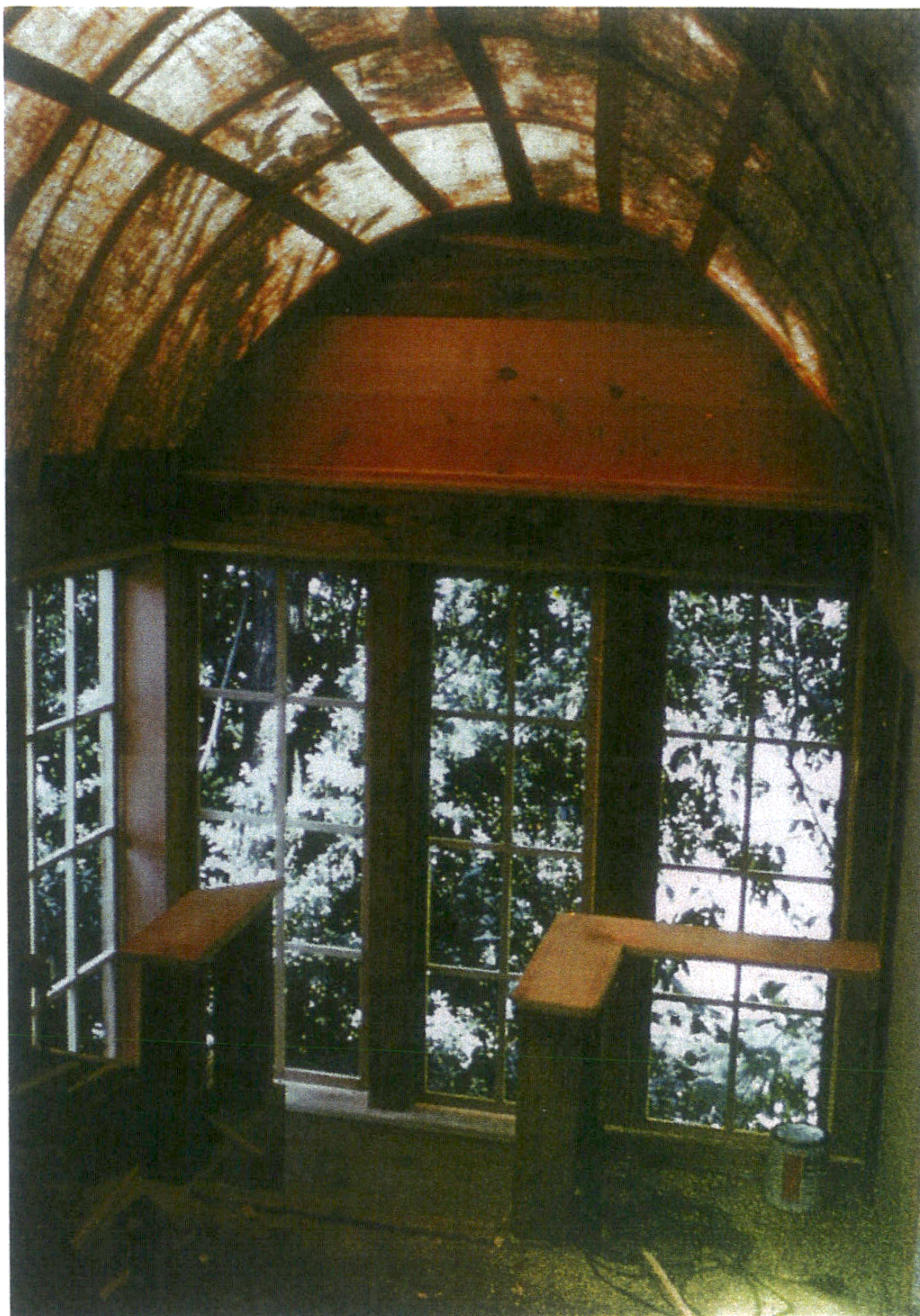
Figure 3: The Experimental Cottage at the CES, based on APL building patterns
