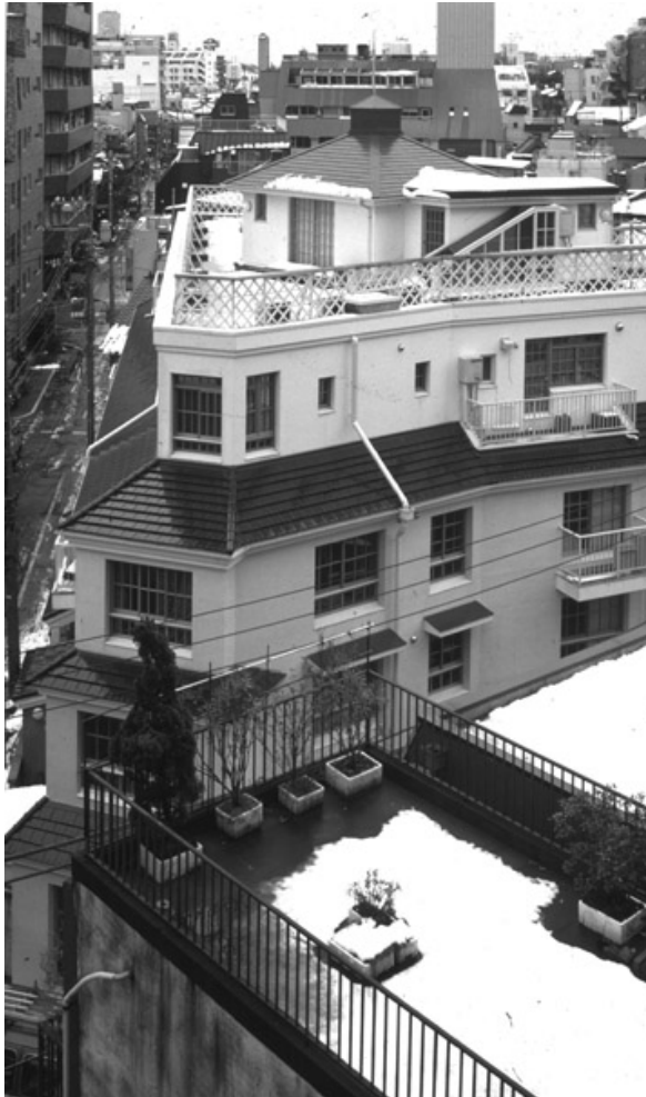
Figure 15 The completed Emoto apartment building
