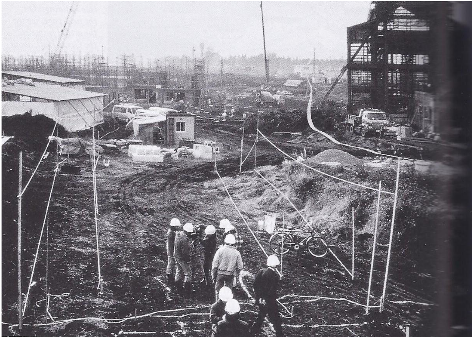
(Page 194) We are using this to illustrate the stakes, and poles, and ropes, which allowed us to mark the position of the entrance street. In the picture we see several of our crew laying out the detailed position of the entrance street, with the long stakes and ropes, all the time judging the shape and position of the space of the entrance street as it was developing
