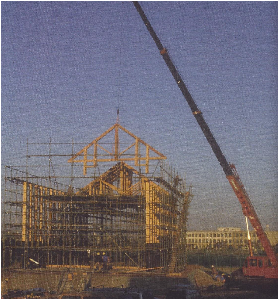
(Page 280) Erection of the Judo Hall in early morning light
