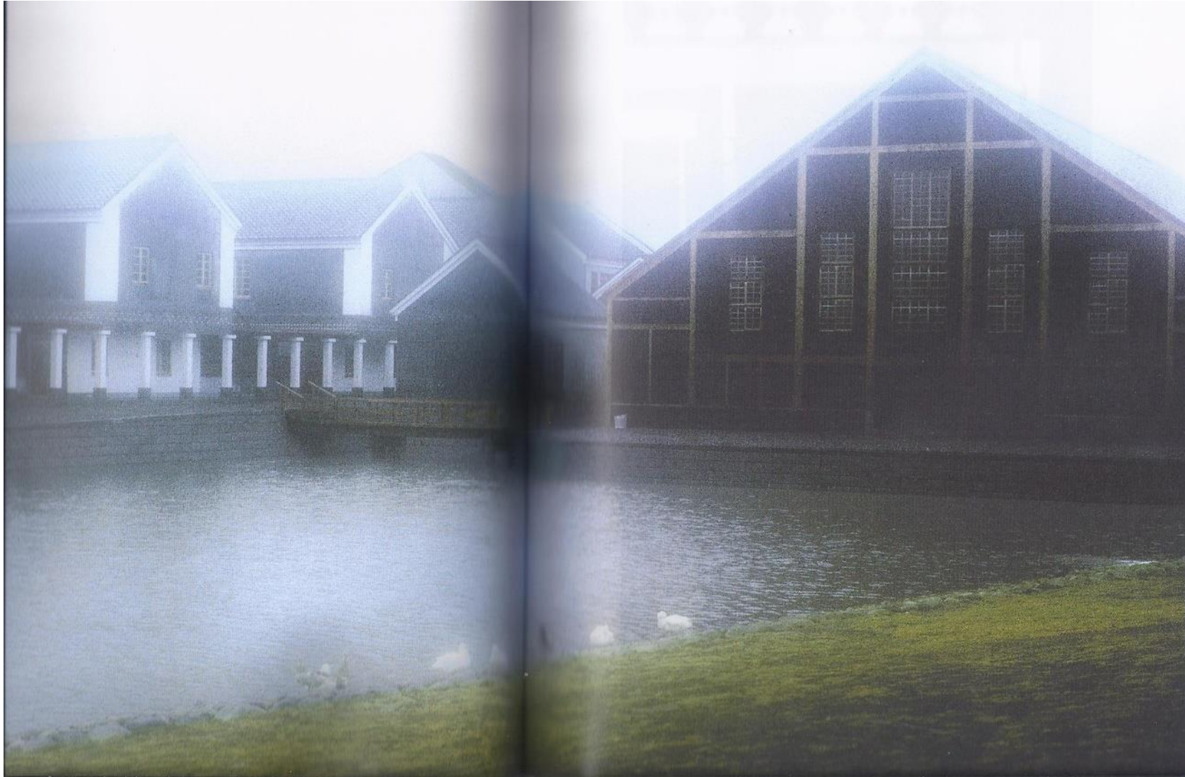
The gymnasium is finished in kura shikkui (black plaster) and one of the Homebase Streets is fully visible. Peeping over the roofs of the Homebase Street, the high roof of the Central Building may be seen in the further distance
