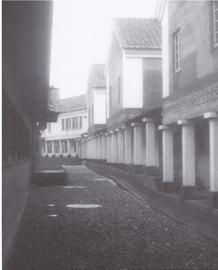
(Page 33) Interior colonnaded street within the campus
