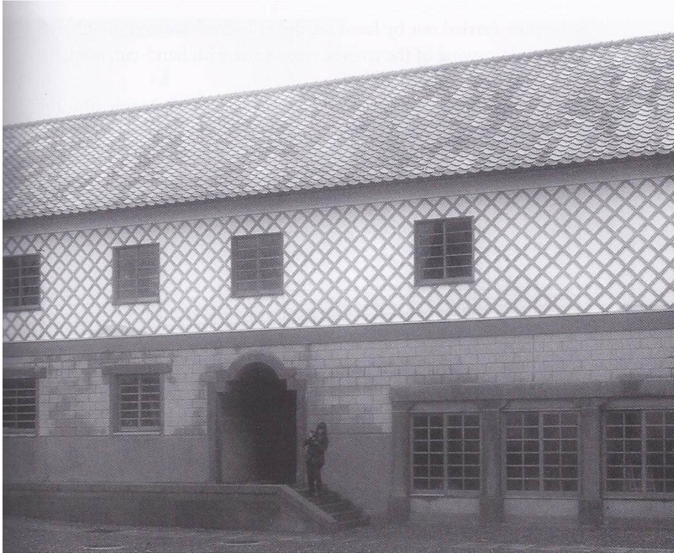
(Page 29) The second storey wall is a trellis of fine concrete splines, with the spaces between the splines plastered in white
