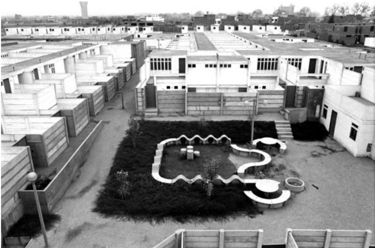
Plaza at south end of cluster with play and social area. Note ramp on left, up to higher level access street between houses. Long units on left and one pair of short units in middle, at end of row.
