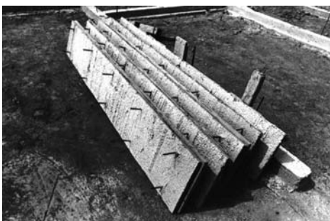
Completed panels with distance pins. Paneles terminados con pernos espaciadores.
