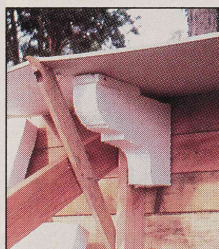
T he children's bedroom (left), and (below) a styrofoam and plywood bracket experiment and the final, poured concrete version that holds up the second-story bay.
