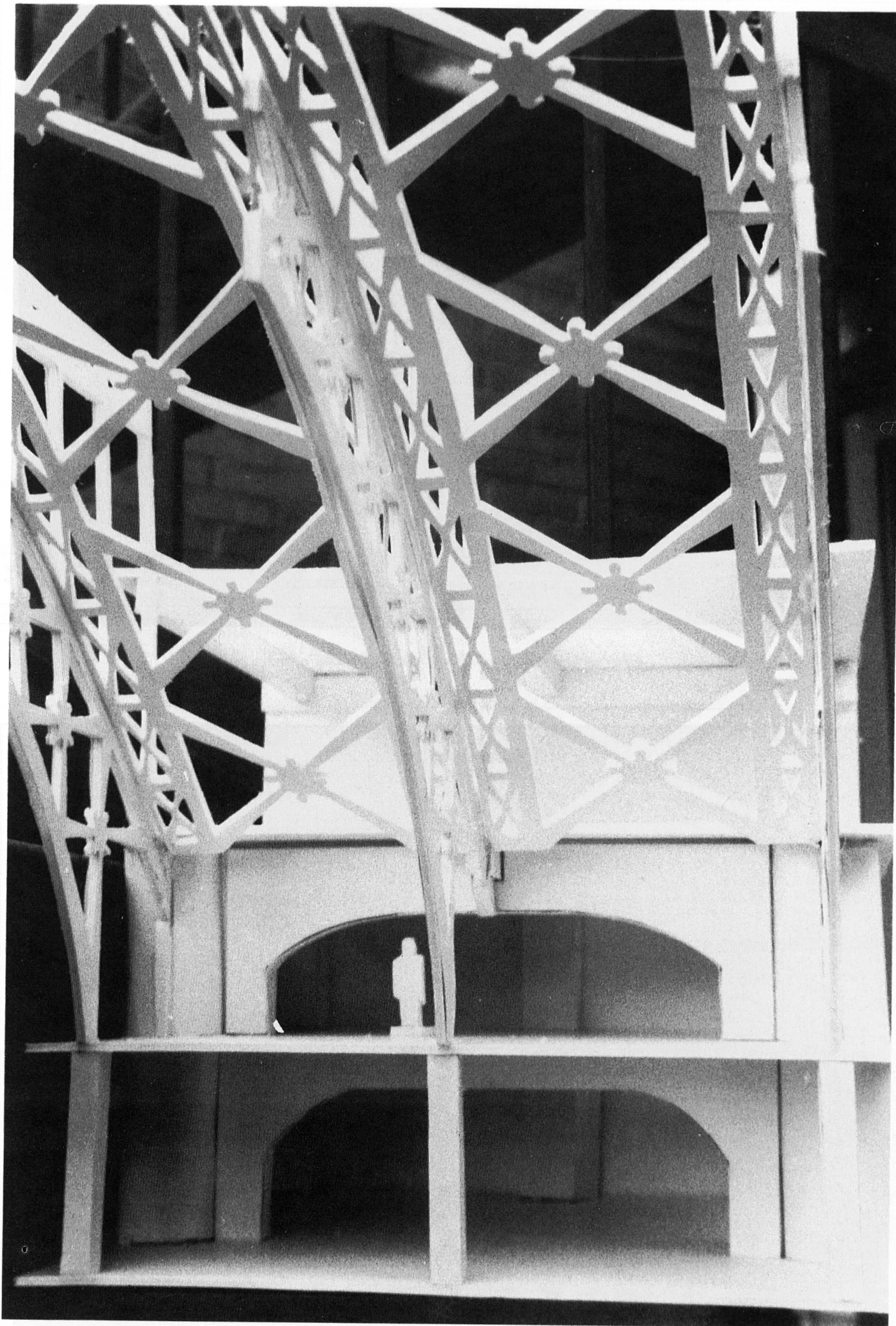
Another view of X-bracing and longitudinal arch system
